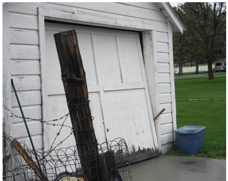
Karen Frandsen’s neighbor ran a pesticide business out of his residential home. These photos, taken by Ms. Frandsen, show the shed and the unmarked containers strewn about on the property, with no signs indicating that pesticides were being stored, mixed, or dumped.
